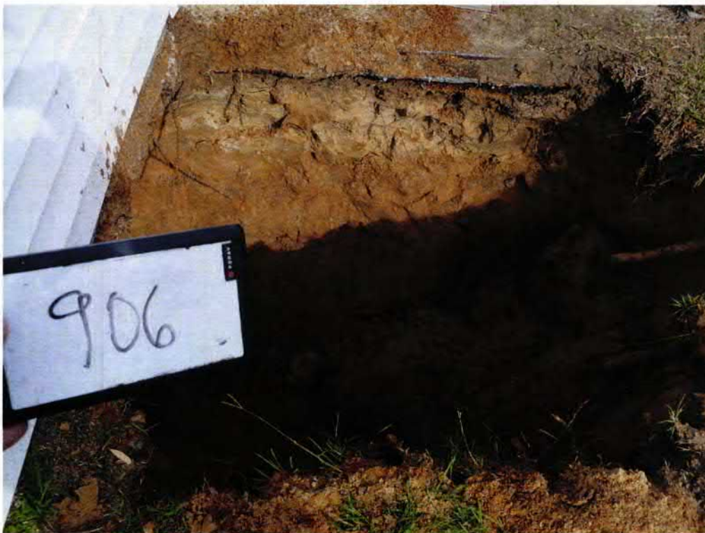
Picture 2: UST 906Barracuda excavation.
